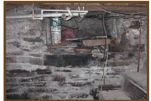
Sealed up tunnel in the cellar. Ted Zendarski, Photographer
